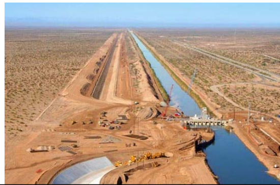
All-American Canal lining project
